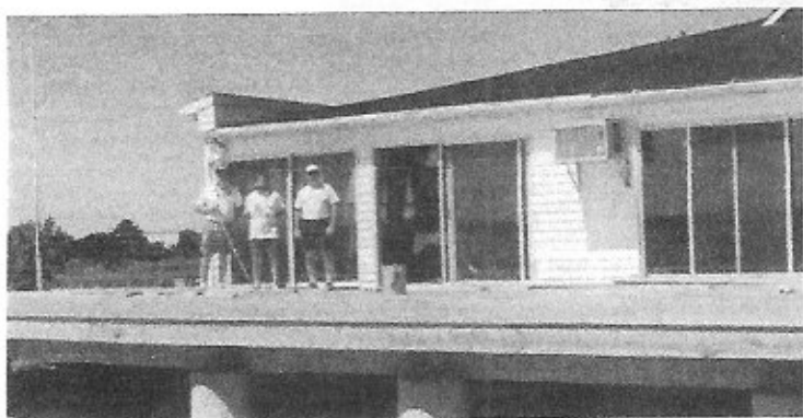
The New Deck
