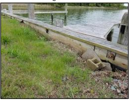
Figure 4. NE Section of Bulkhead - Spring 2016 - showing one area of washout
