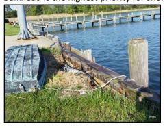
Figure 5. SW section of bulkhead - Spring 2016 - showing shore washout and deteriorating timber and hardware
